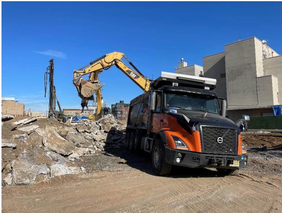
Photo 2: View of contractor loading C&D in Lot 14, facing north.
