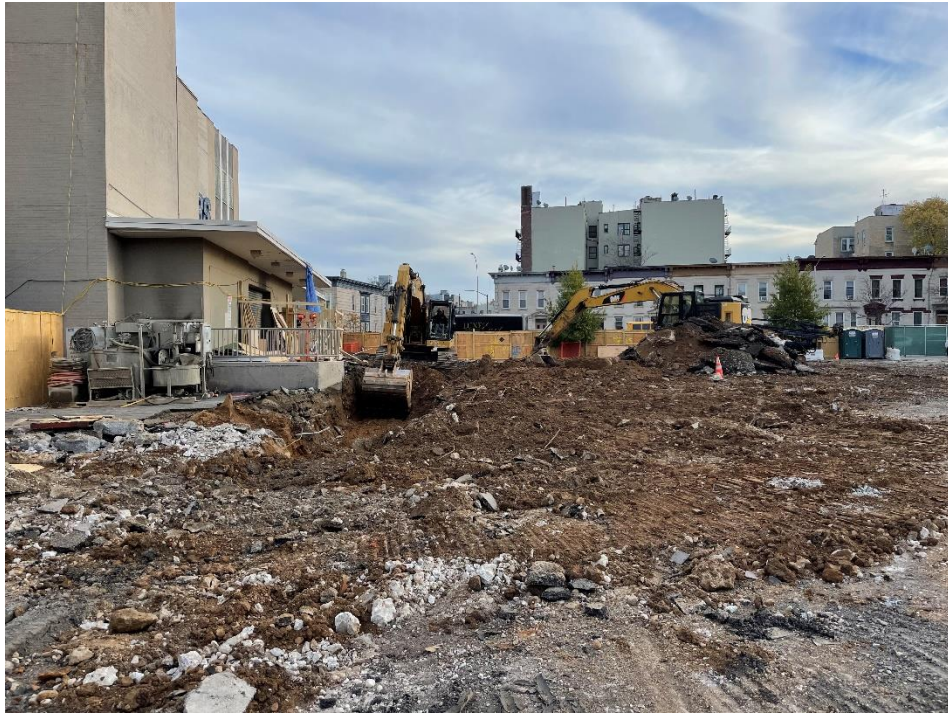
Photo 1: View of contractor grading Site soils in Lot 14, facing south.
