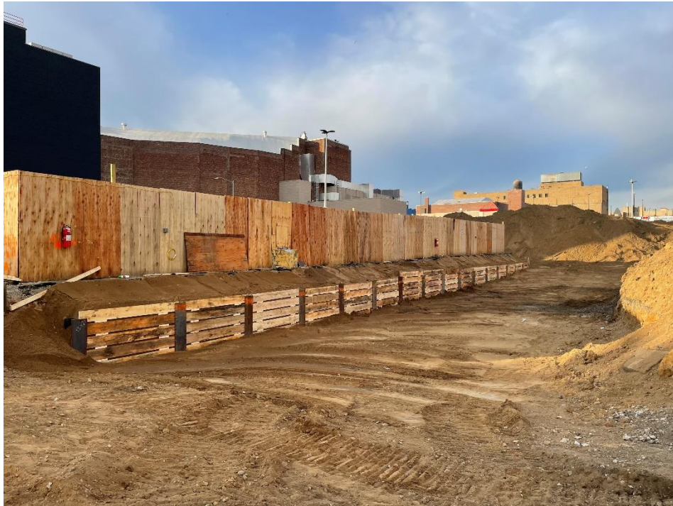
Photo 1: View of H piles and lagging installed in Lot 14, facing north-northwest.
