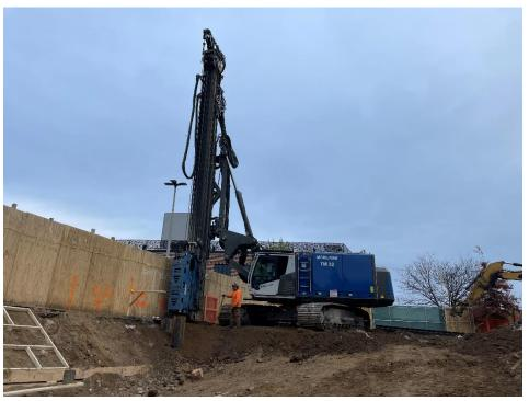
Photo 1: View of contractor installing H piles in Lot 14, facing northeast.
