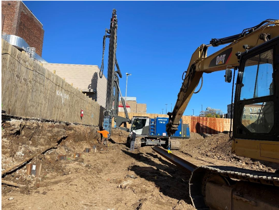
Photo 1: View of contractor installing H piles in Lot 14, facing west.
