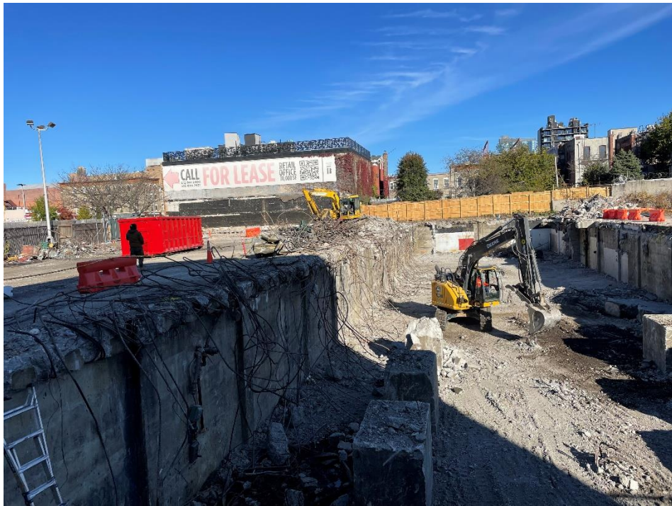
Photo 2: View of contractor stockpiling demo debris from Lot 53, facing north.
