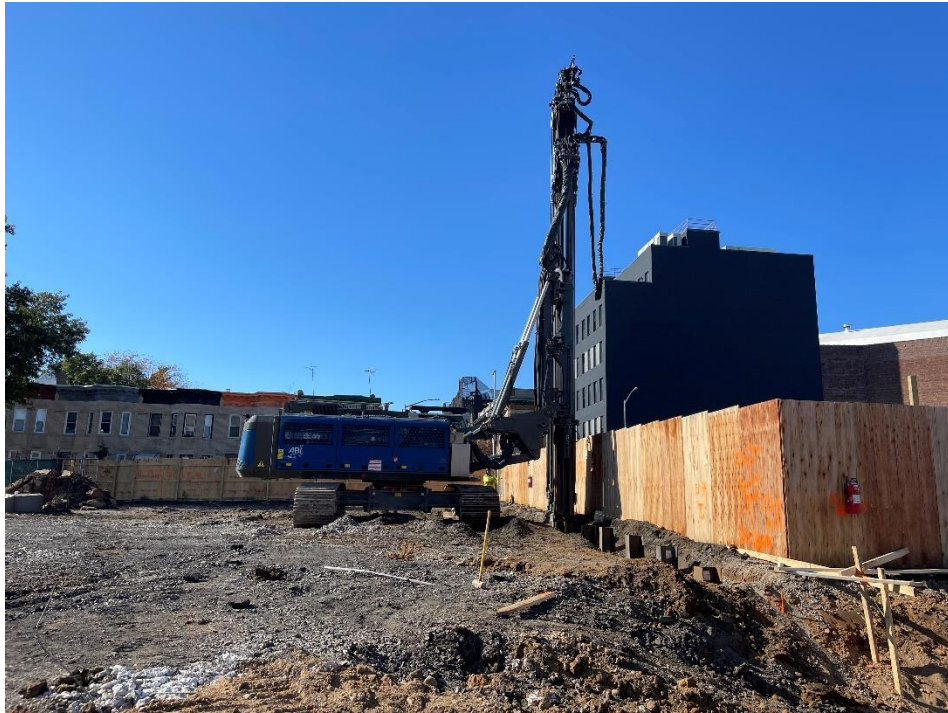
Photo 1: View of contractor installing H piles from Lot 14, facing southwest.
