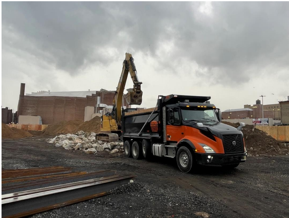
Photo 2: View of contractor loading concrete for disposal from Lot 14, facing northwest.
