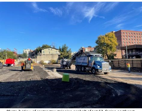
*Photo 2: View of contractor stripping asphalt of Lot 53, facing northeast.*
