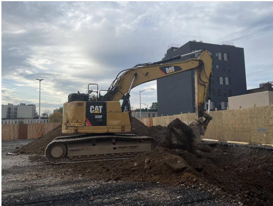
Photo 2: View of excavation for SOE installation along the perimeter of Lot 14, facing southwest.
