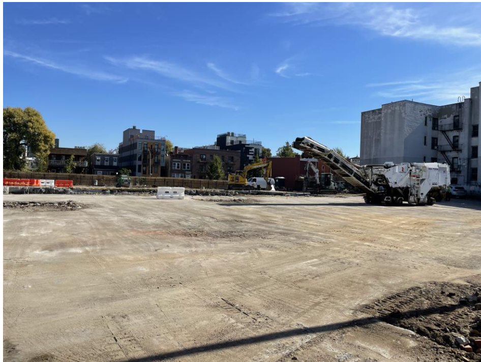
Photo 2: General view of the Site, in Lot 53, facing southeast.
