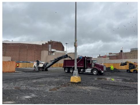
Photo 1: View of asphalt stripping in lot 14, facing northwest.
