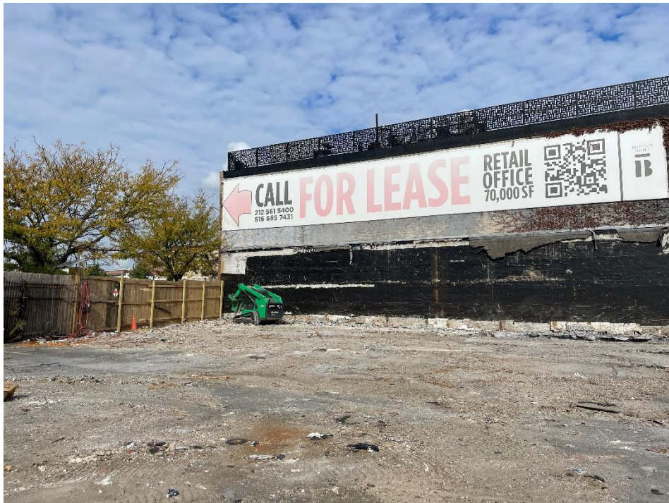
Photo 2: View of demolition work, facing northwest.
