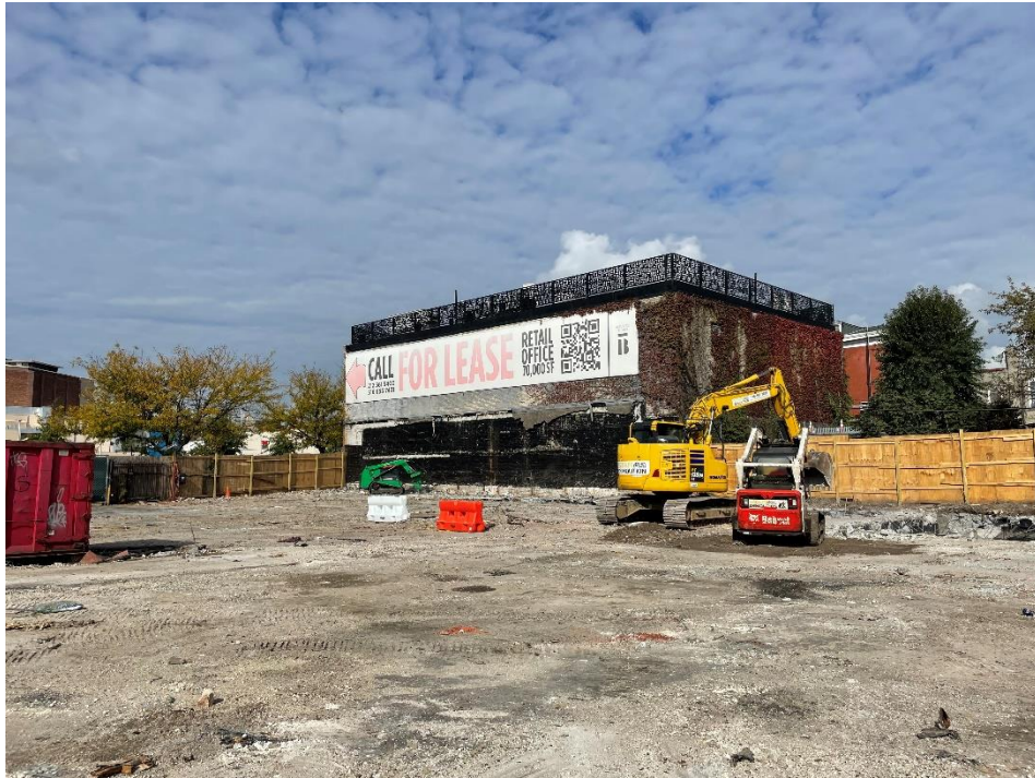
Photo 1: View of demolition work, facing northwest.
