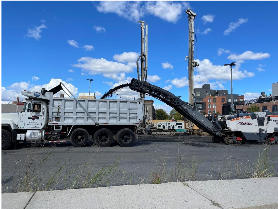
Photo 1: View of asphalt stripping on Lot 14, facing north.
