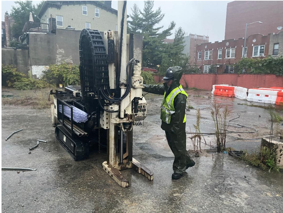
Photo 1: View of soil drilling activities, facing east.
