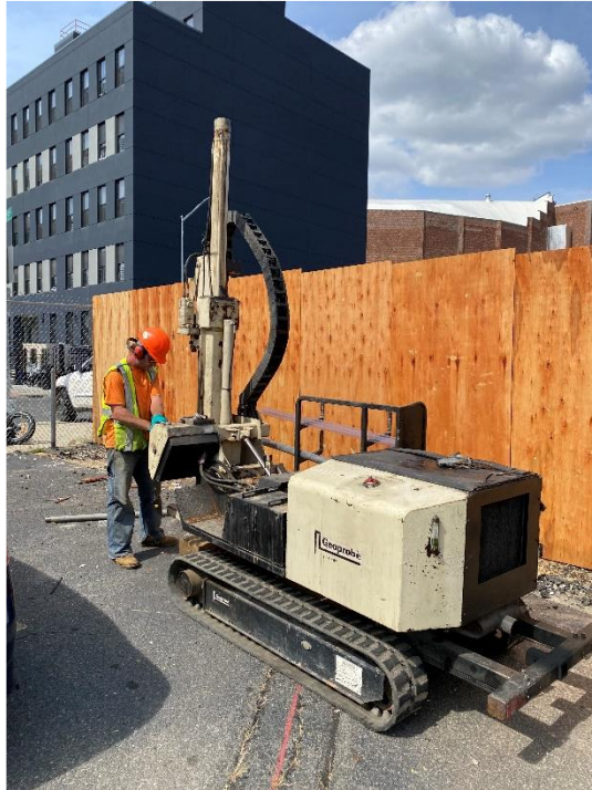
Photo 1: View of contractor advancing waste characterization borings, facing west.
