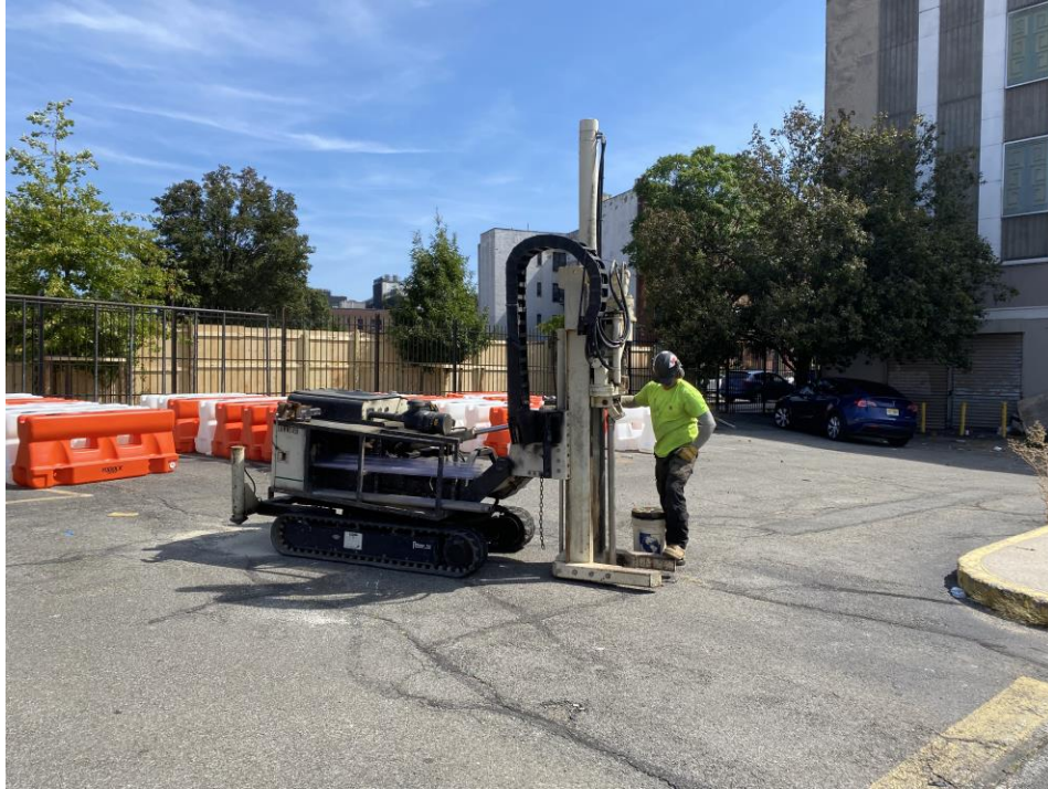
Photo 1: View of contractor advancing waste characterization borings, facing southeast.
