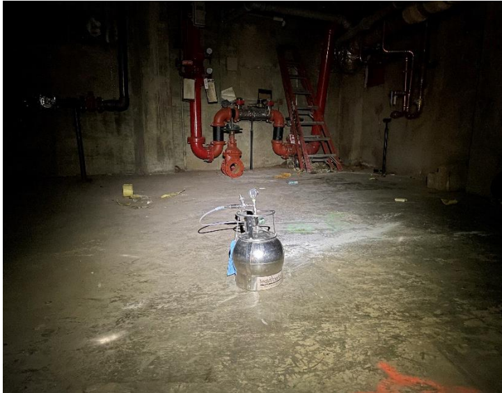
Photo 2: View of sub-slab soil vapor sampling activities, facing west.
