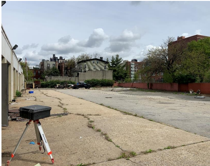
Photo 2: View of Site activities, facing north-northeast.
