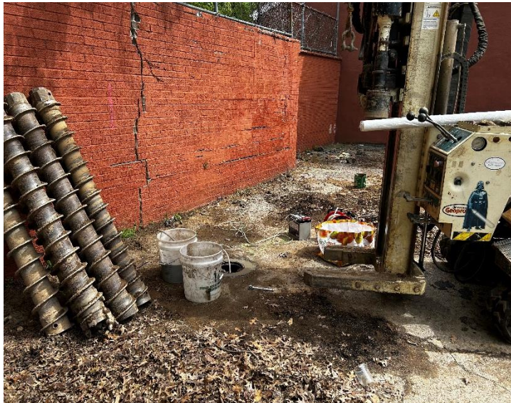
Photo 2: View of monitoring well development, facing south.
