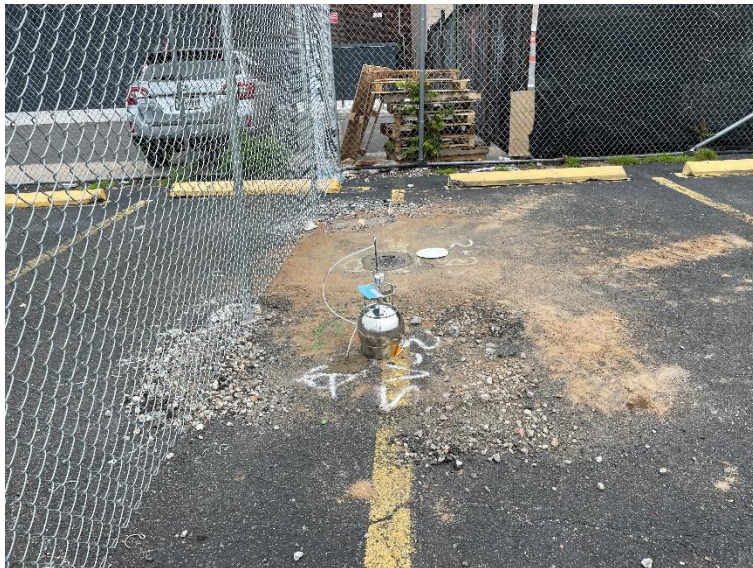
Photo 2: View of soil vapor sampling, facing west.
