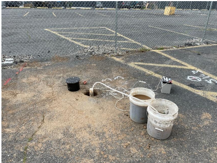
Photo 2: View of monitoring well development, facing west-northwest.
