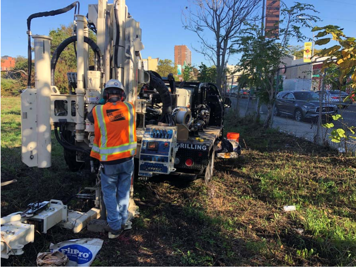
Photograph No. 1: Representative photograph of soil boring installation at the Site.
