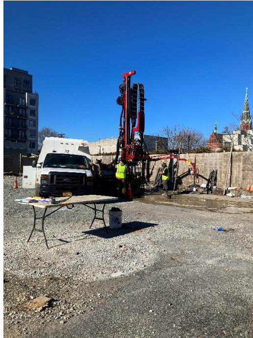
Photo 1: View of Coastal advancing boring on SB-3_W.
