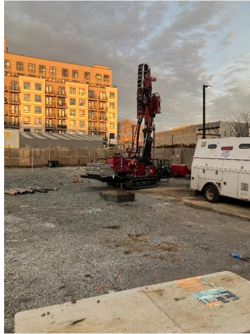
Photo 1: View of Coastal advancing a boring at SB-3_W1.
