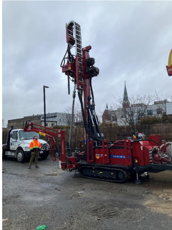
Photo 1: View of Coastal advancing boring on SB-10.
