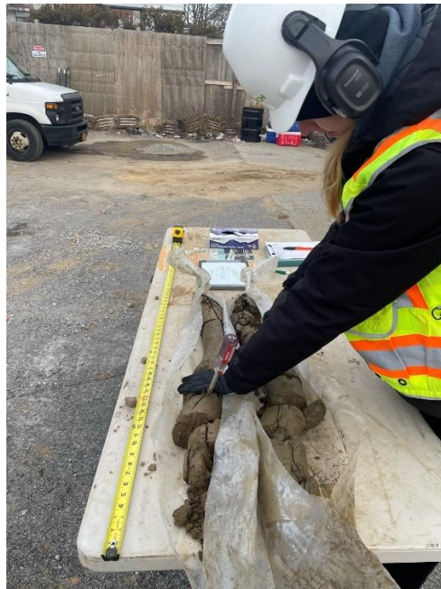
Photo 2: View of HA collecting PID readings from SB-3_W (depth: 15-20 ft bgs).
