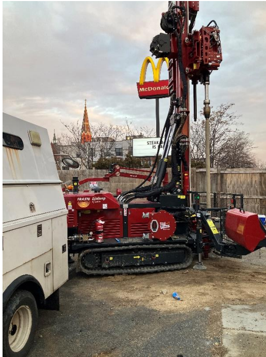
Photo 1: View of Coastal advancing boring on SB-3_E2.
