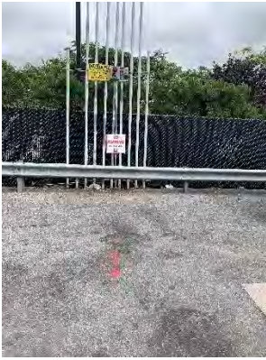
Picture 1: AUTO SHUT OFF ELECTRICAL LINES.
