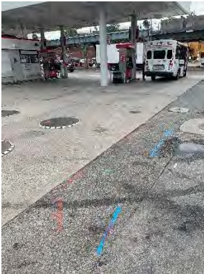
Picture 3: WATER AND ELECTRICAL LINES GOING TO THE BUILDING.
