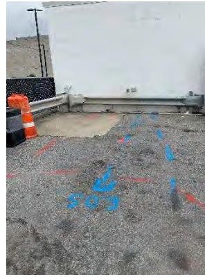
Picture 2: SIGNAL OF WATER LINE WAS LOST AND PICKED UP AGAIN NEAR THE BUILDING.
