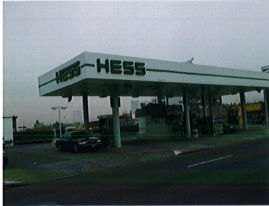
Looking northeast at Station
