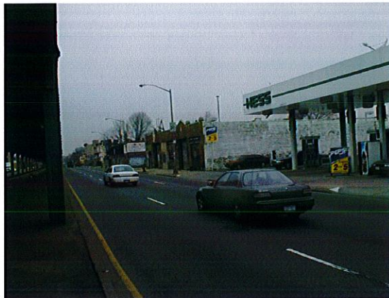
Looking west at Station and Commercial buildings
