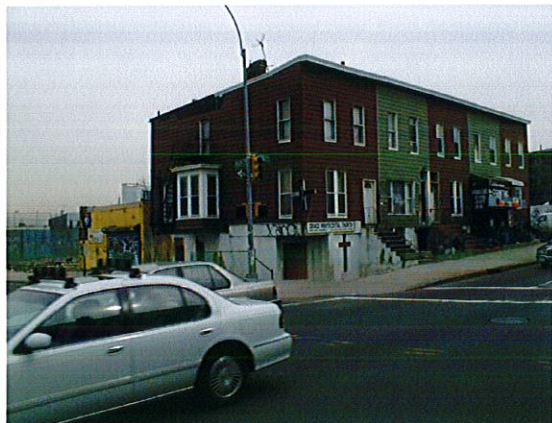
Looking east from Station at Church
