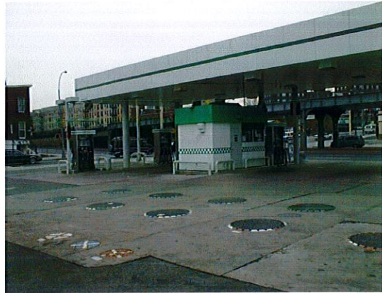
Looking southeast at rear of Station
