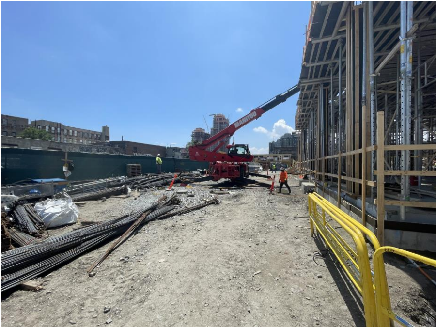
Photo 1: General view of the Shore Public Walkway (SPW) (facing southeast)
