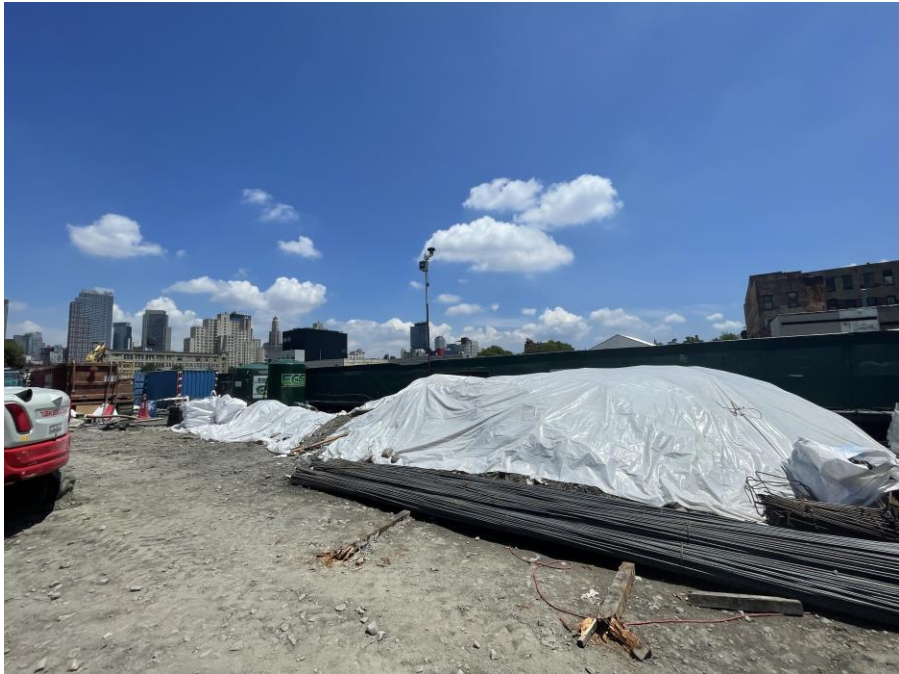
Photo 2: View of stockpile covered with polyethylene sheeting within the SPW (facing northeast)
