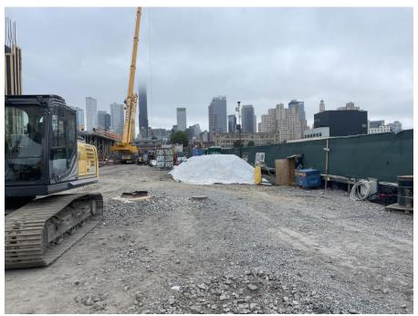
Photo 2: View of stockpile covered with polyethylene sheeting within the SPW (facing north)
