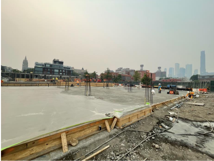
Photo 1: General view of Society Brooklyn during concrete slab installation (facing north)
