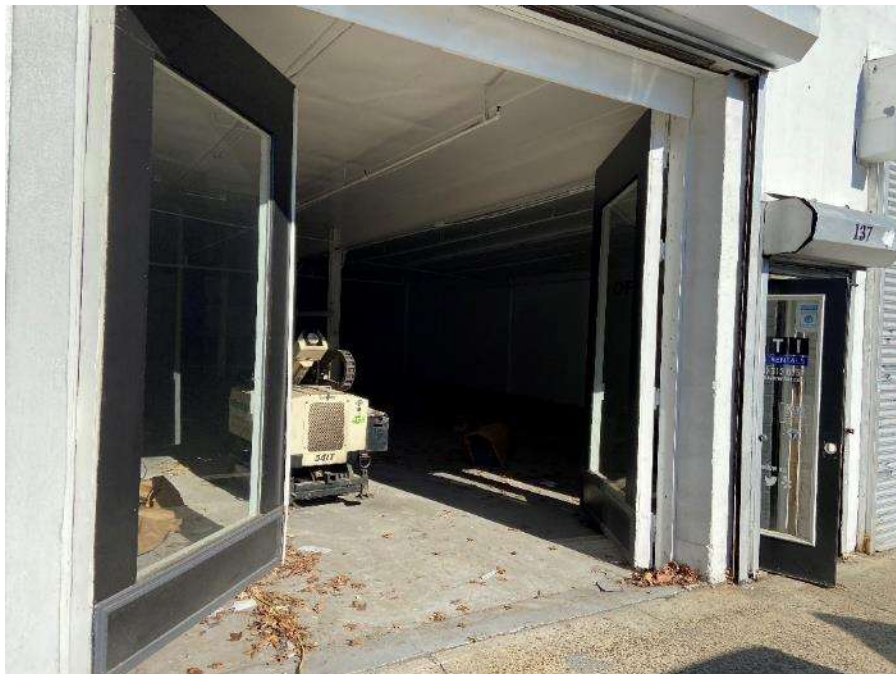
Photo 2: Eastern advancing soil boring SB23 (facing northeast).
