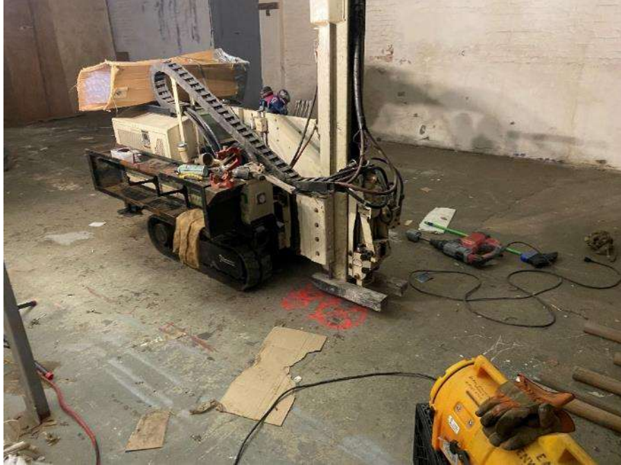
Photo 1: Eastern advancing soil boring SB21 (facing northeast).
