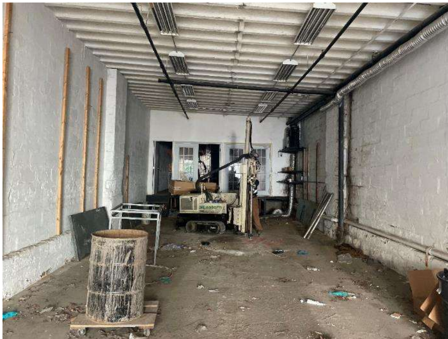
Photo 2: Eastern advancing soil boring SB17 (facing southwest).
