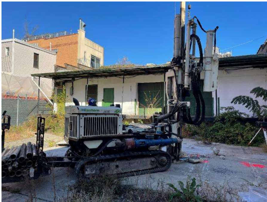
Photo 2: Eastern advancing soil boring SB15 (facing north).
