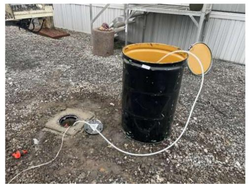
Photo 1: AARCO developing monitoring well couplet MW15-N1 (facing north).
