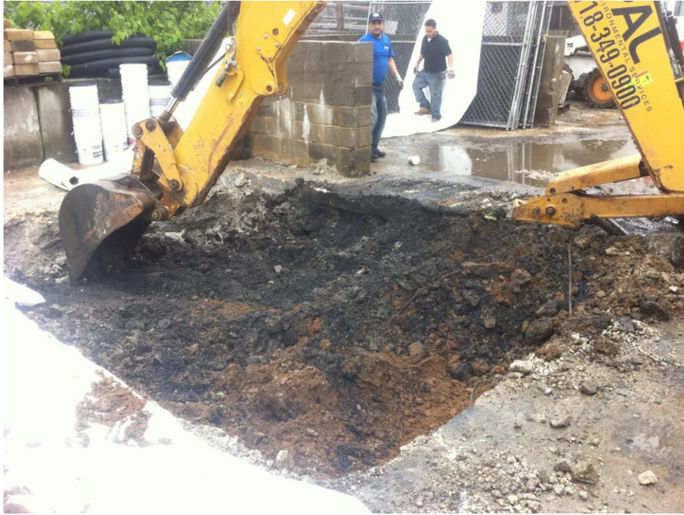
Photo 3: View of excavation with concrete removed.
