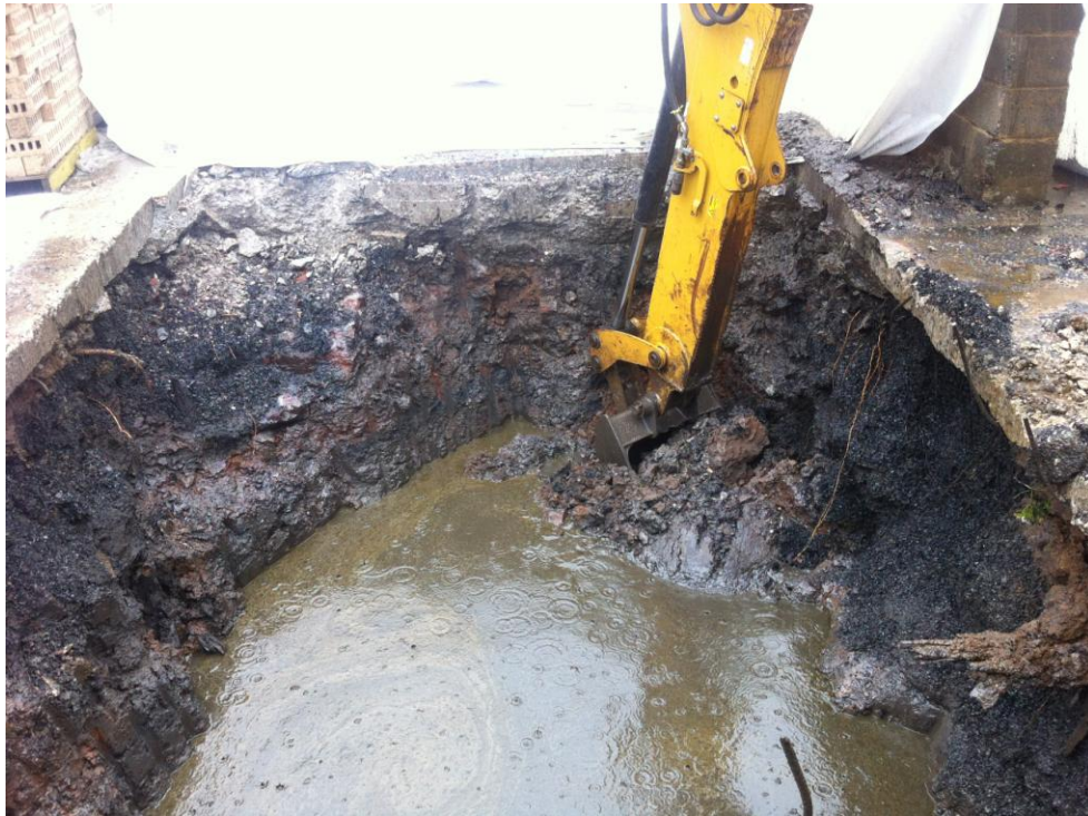
Photo 4: View of excavation of petroleum impacted soil at the water table.
