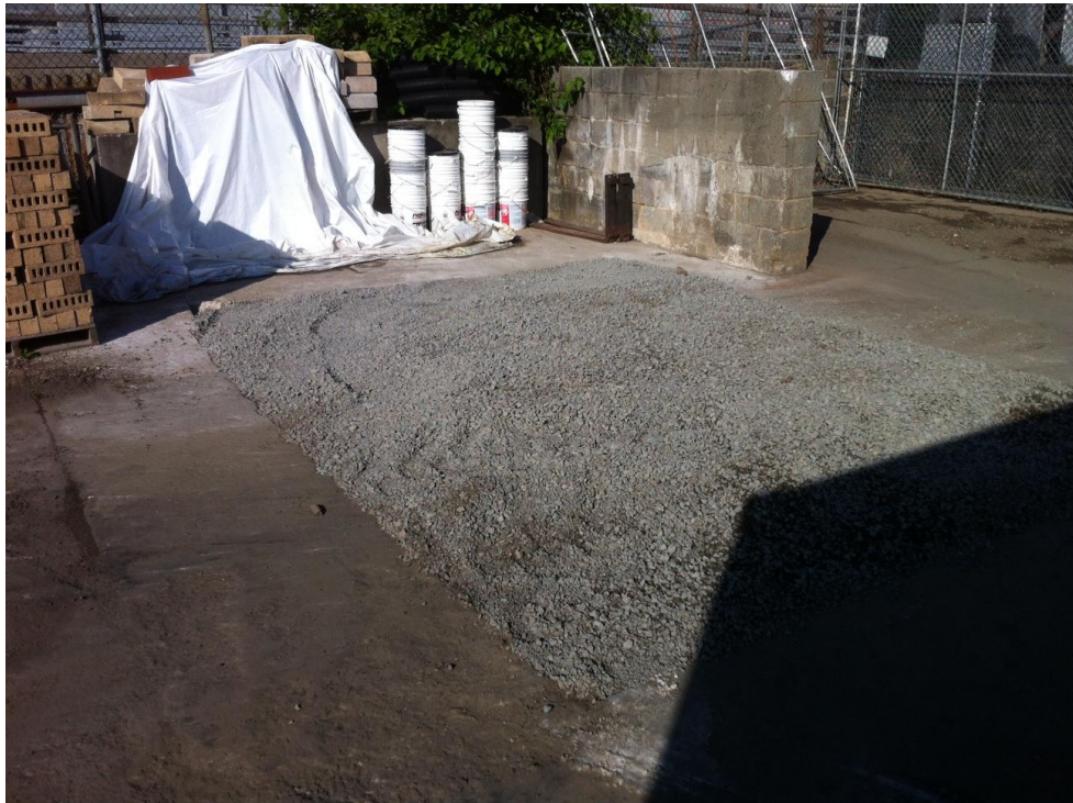
Photo 6: View of backfilled excavation.
