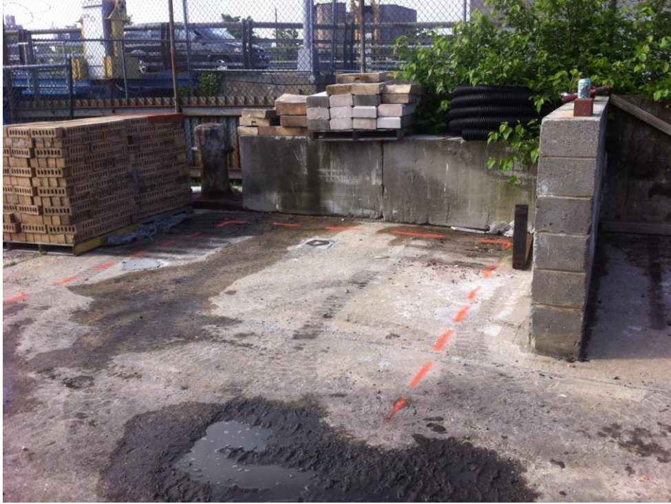
Photo 1: Excavation area prior to concrete removal.
