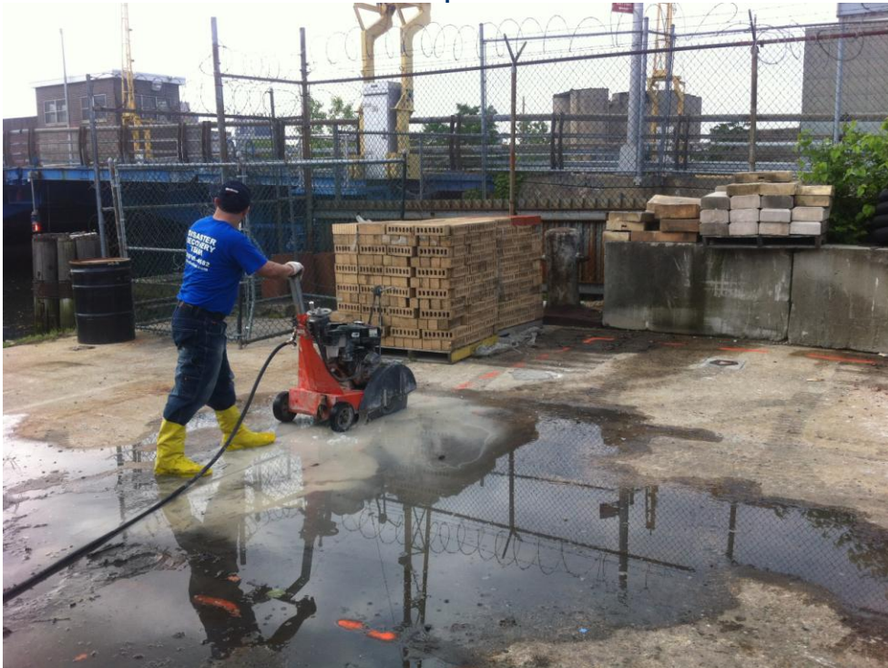
Photo 2: A concrete saw was used to cut out the excavation area.
