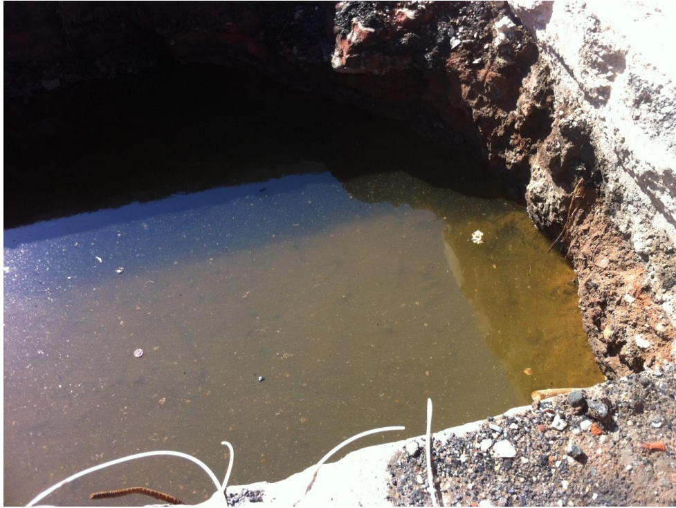
Photo 5: View of clean water in the excavation.
