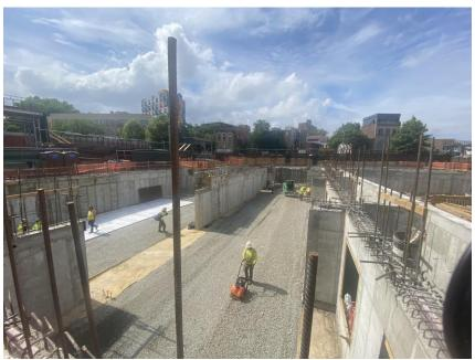
**Photo 2:** View of graded ¾-inch gravel and W.R. Meadows PRECON® waterproofing installed in the western part of the site (facing northwest).
