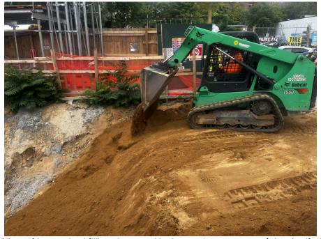
Photo 2: View of Legacy backfilling clean sand in the southeastern part of the site (facing east).
