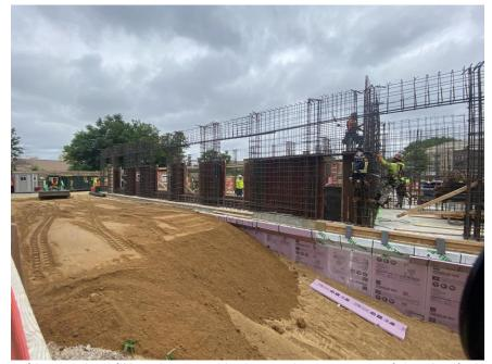
Photo 2: View of Legacy backfilling clean sand in the southeastern part of the site (facing southwest).
