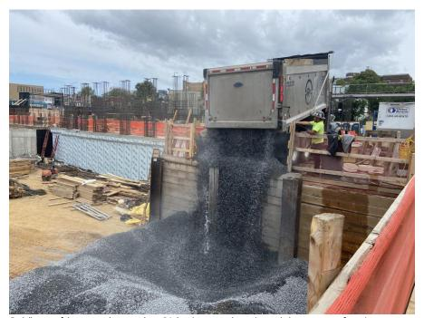
**Photo 2:** View of Legacy importing ¾-inch gravel and applying water for dust suppression in the southern part of the site (facing northeast).
