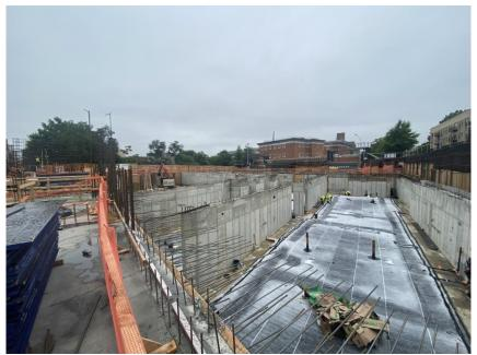
**Photo 2:** View of Legacy installing W.R. Meadows PRECON® waterproofing atop ¾-inch gravel in the northern part of the site (facing southwest).
