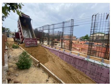
Photo 1: View of Legacy importing clean sand for backfill in the the eastern part of the site (facing southwest).
