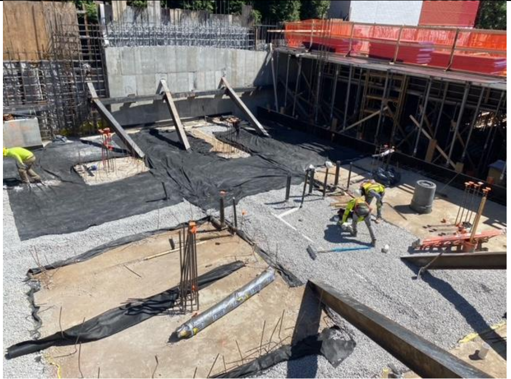
Photo 2 – Facing North Laydown of geotextile fabric over clean stone/piping.
