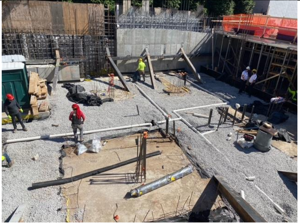
Photo 1 – Facing North Plumbers installing SSDS piping/riser.
