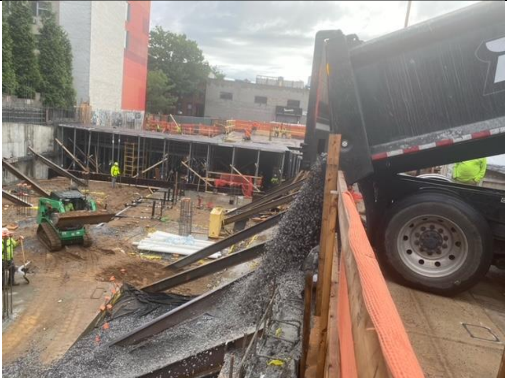
Photo 2 – Facing East Receive one load of clean 3/4" stone for SSDS.
