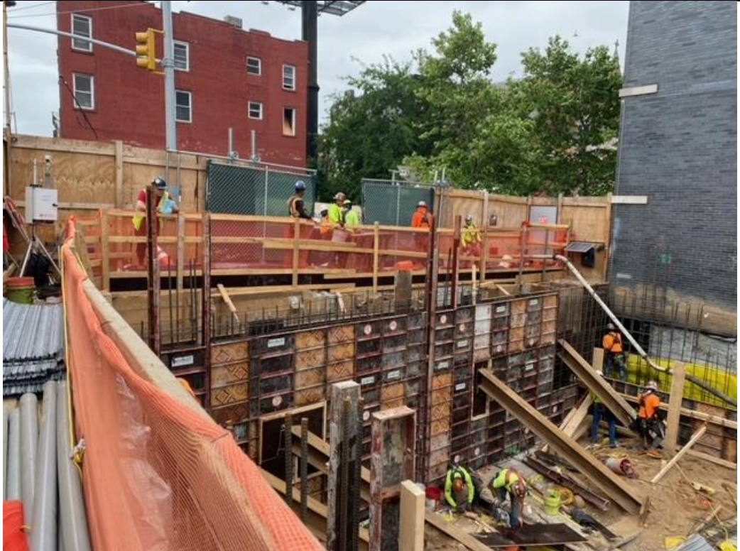
Photo 2 – Facing Northeast Installation of forms along western wall.
