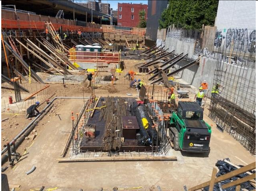
Photo 1 – Facing West General cleanup final piping of East slab.
