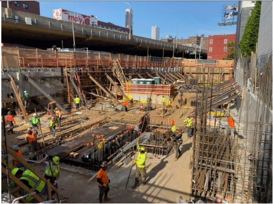
Photo 4 – Facing Southwest Cleanup along eastern slab.
