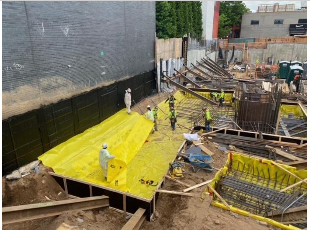
Photo 2 – Facing Northeast Installation of Stego vapor barrier along northern footer.
