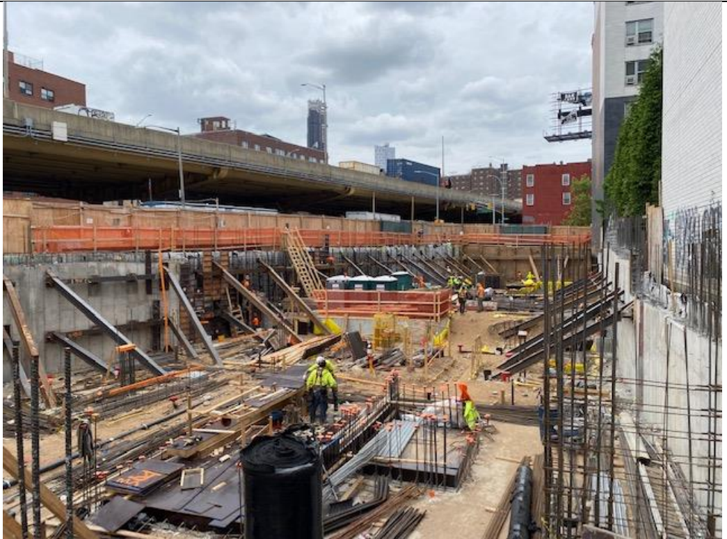
Photo 4 – Facing Southwest View of Site from NE corner.
