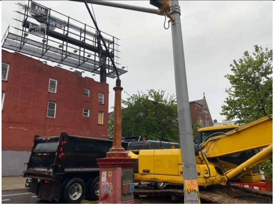
Photo 2 – Facing West Final 2 loads of soil shipped offsite to Coplay facility.
