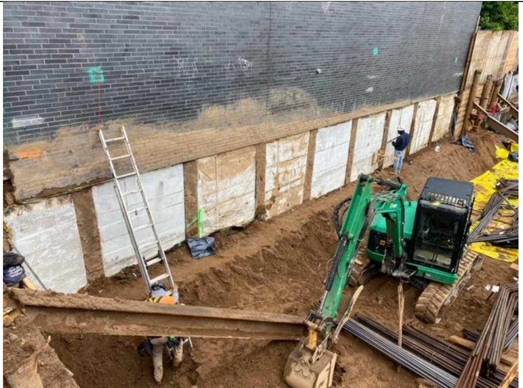
Photo 3 – Facing West Soil grading by footer along western portion of the Site.
