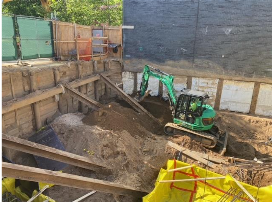
Photo 2 – Facing North Final grading of soil along western wall.
