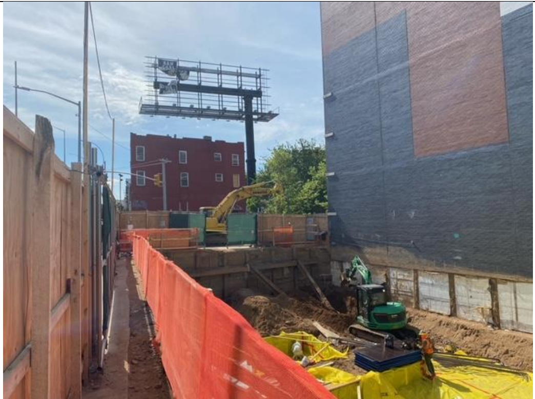
Photo 4 – Facing Northwest Excavator grading soil to stockpile for disposal.
