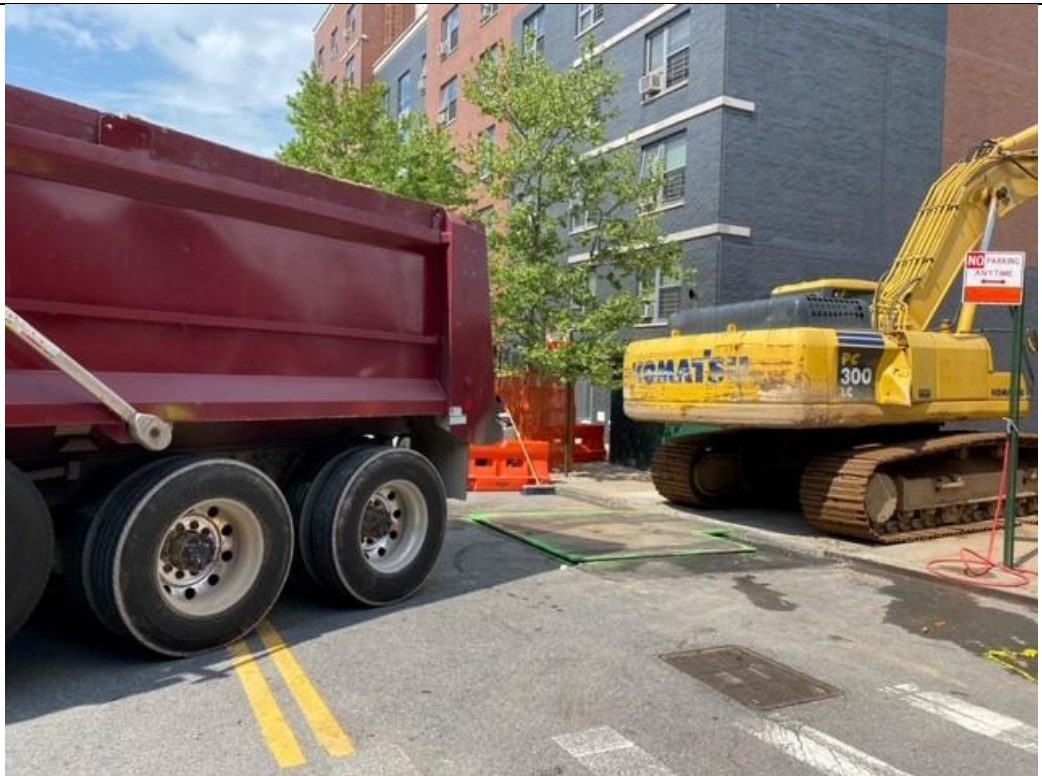
Photo 4 – Facing Northeast Truck backing up to export soil to Coplay Quarry Facility.
