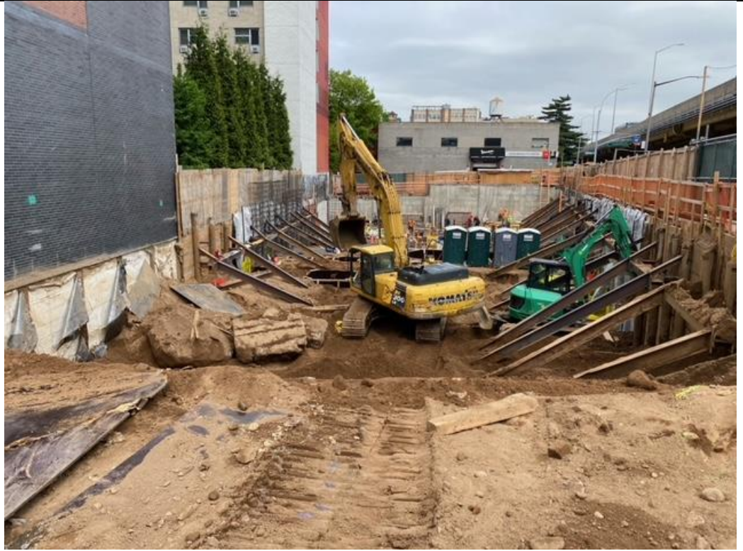
Photo 1 – Facing East Grading soil along rakers and walers.
