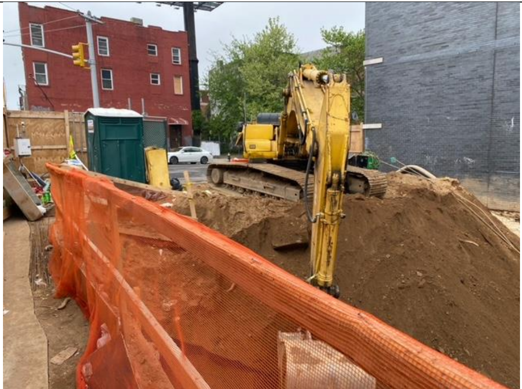
Photo 4 – Facing Southwest CAMP 1 station located near stockpiled soils along entrance gate.
