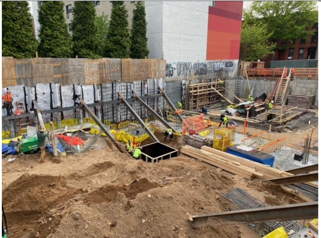
Photo 4 – Facing Northeast Waterproofing installation along NE lagging.
