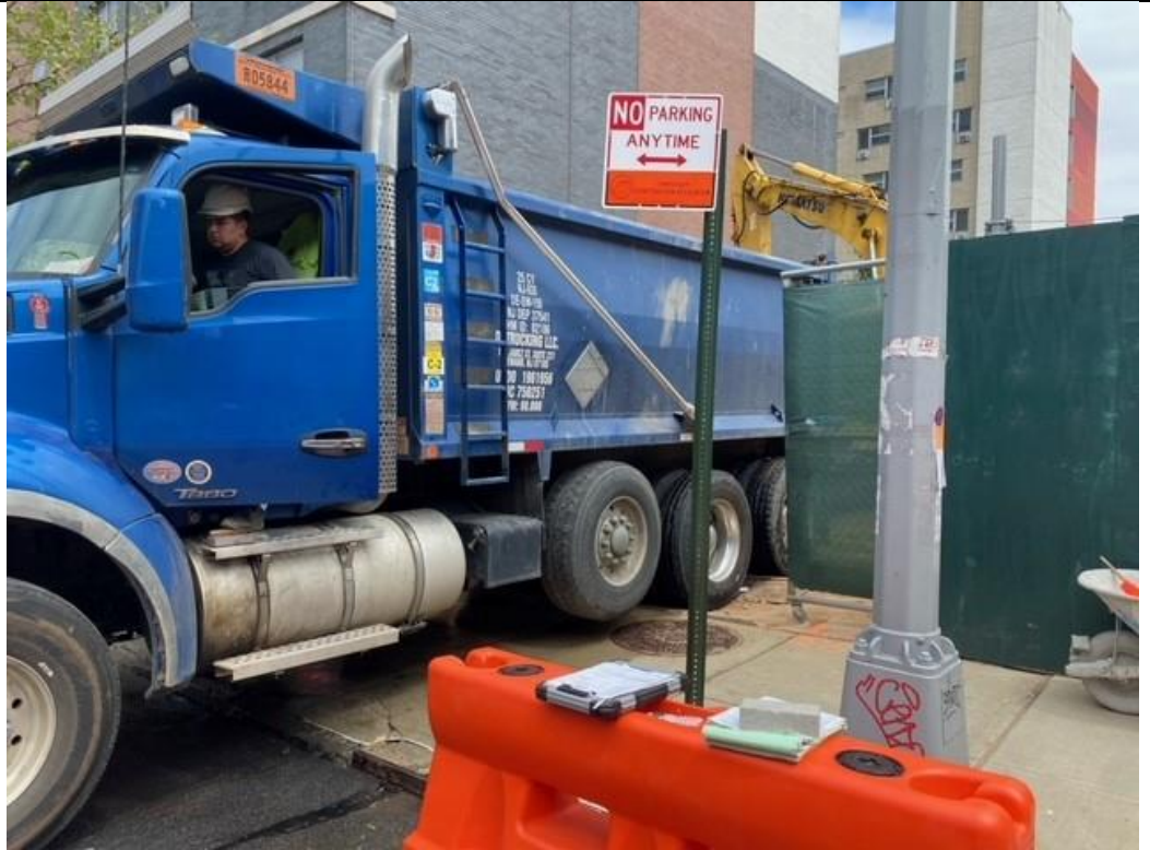
Photo 1 – Facing West Excavator loading soil on sidewalk.
