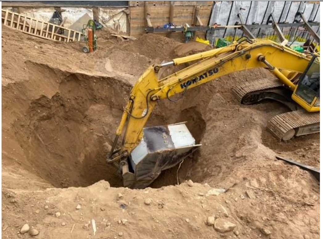
Photo 4 – Facing North Excavator placing the final heel block.
