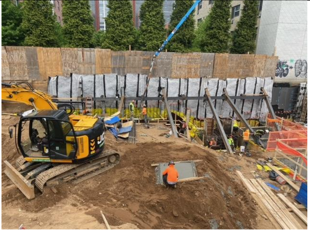
Photo 1 – Facing North Pouring concrete along northern wall.
