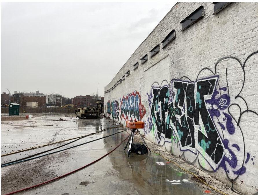
Photo 2: Regensis applying remedial products at injection point IP19 (facing north).
