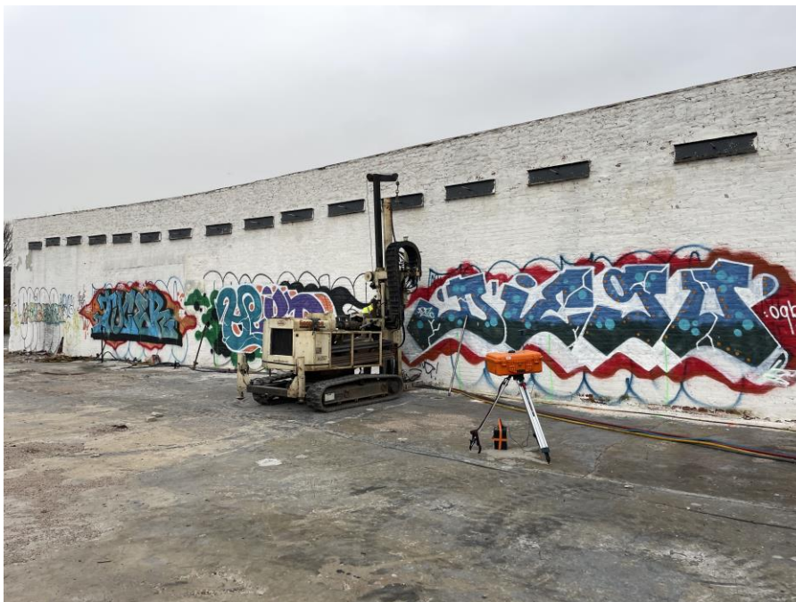
Photo 2: Regensis applying remedial products at injection point IP25 (facing north).
