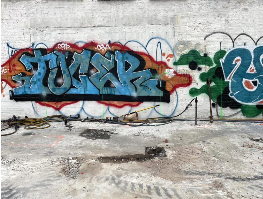
Photo 1: Regensis applying remedial products at injection points IP19 and IP21 (facing north).
