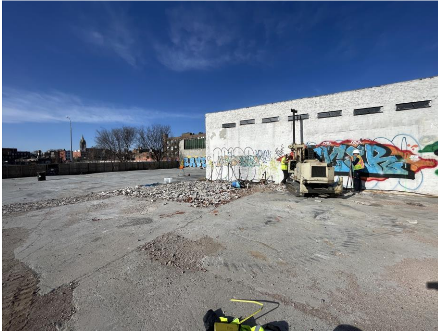
Photo 1: Regensis applying remedial products at injection point IP18 (facing north).
