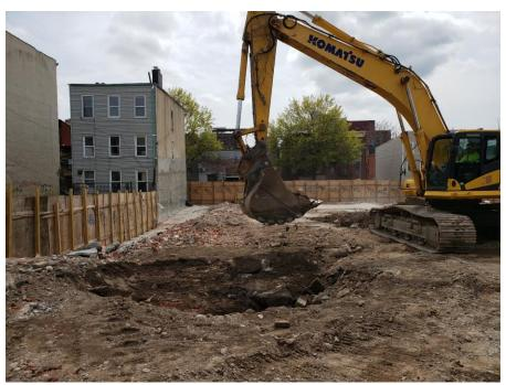
**Photo 1:** Kingdom backfilling an area around a pile cap in the eastern part of the site (facing south).
