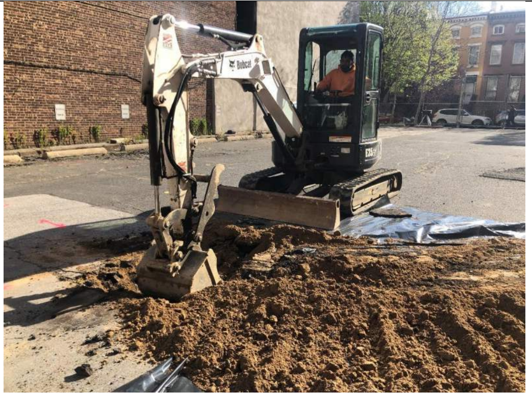
Photo 3 – Backfilling test pit TP-6, facing northwest.
