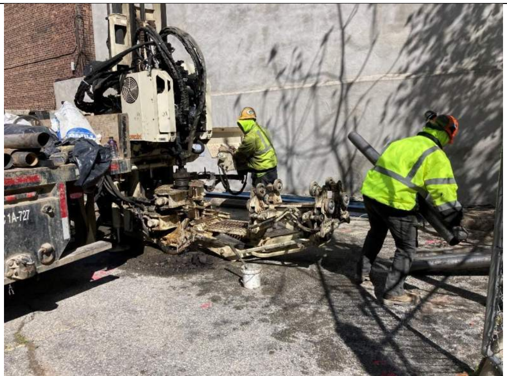
Photo 2 – Drilling at LSB-5, facing northwest.
