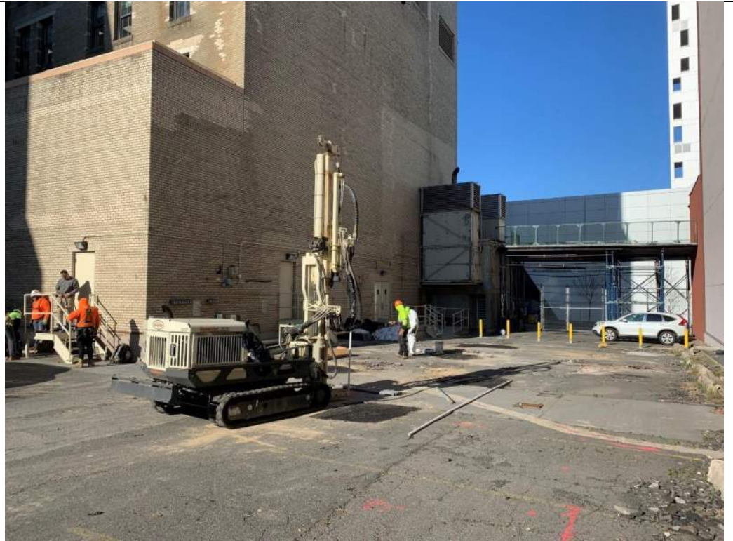
Photo 1 – Drilling at LSV-4A/B, facing west.
