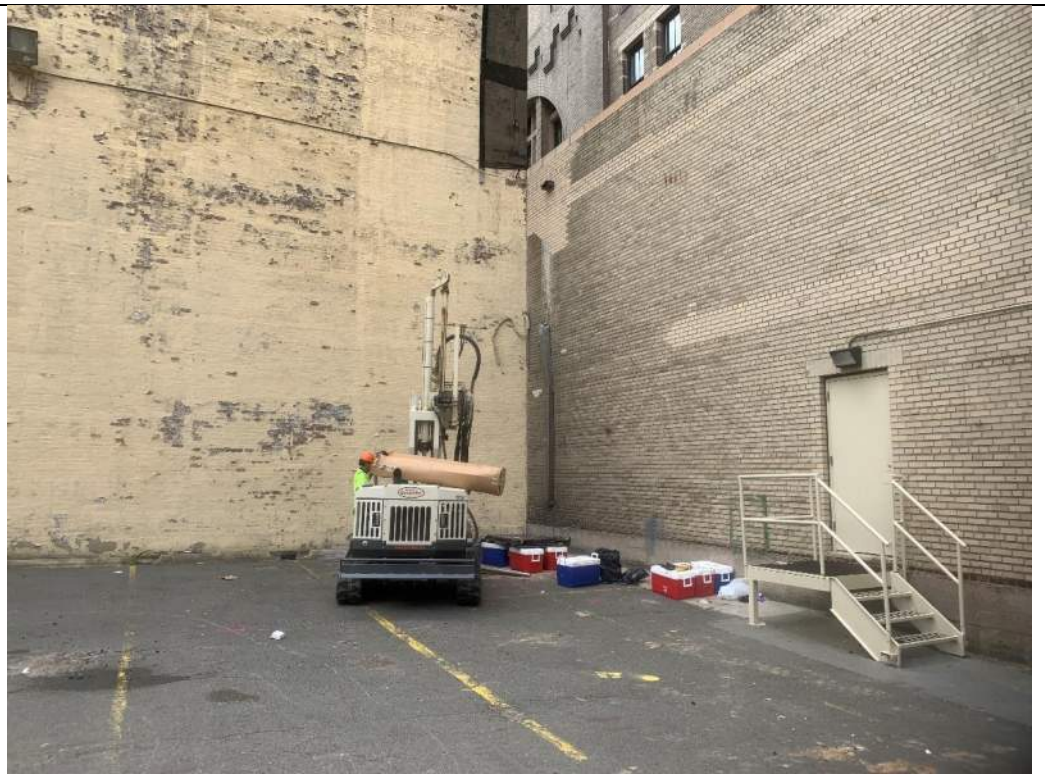
Photo 2 – Drilling at LSB-7, facing southwest.
