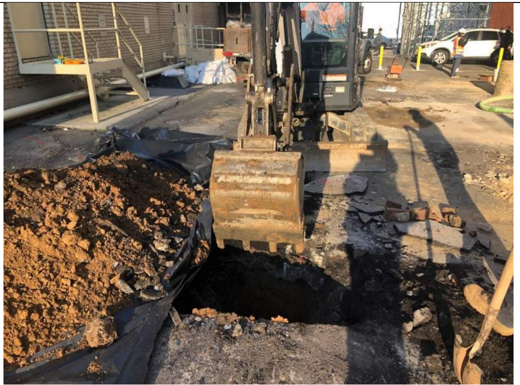
Photo 2 – Excavation of test pit TP-4, facing east.
