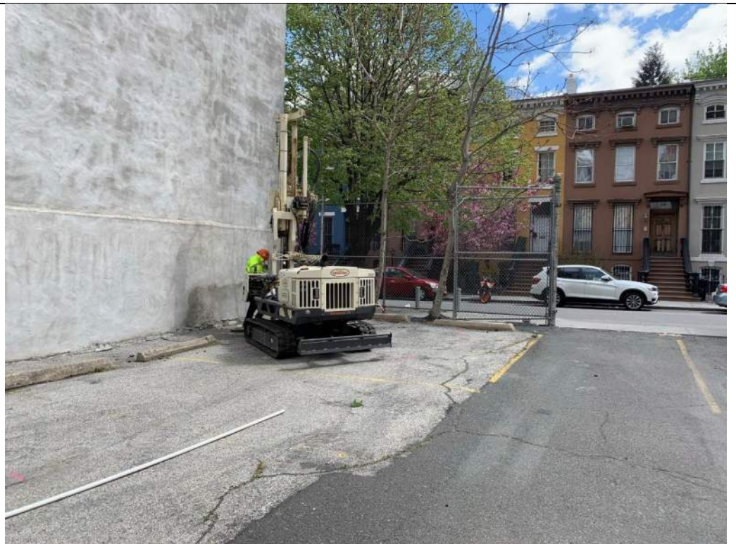
Photo 2 – Drilling at LSV-6A/B, facing northwest.
