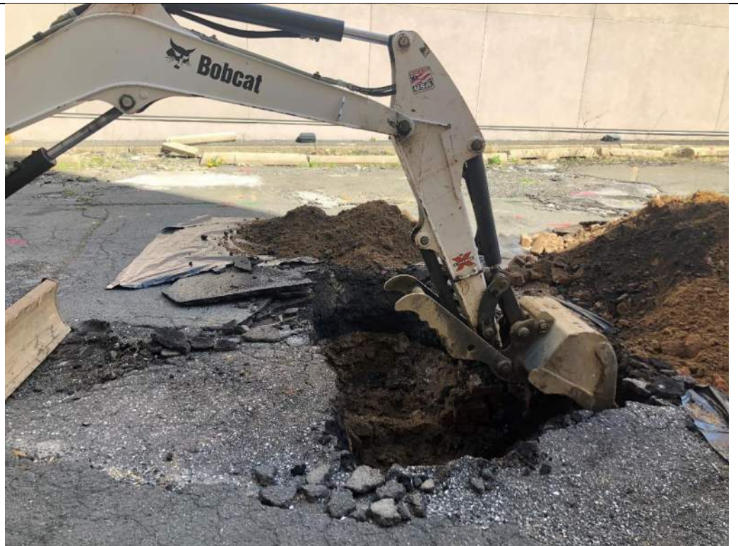
Photo 2 – Excavation of test pit TP-1, facing north.
