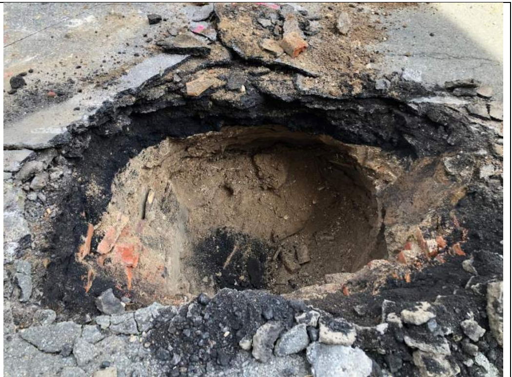
Photo 3 – View of test pit TP-2, facing south.
