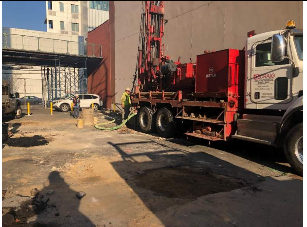
Photo 1 – Geotechnical drilling at LB-1, facing northeast.
